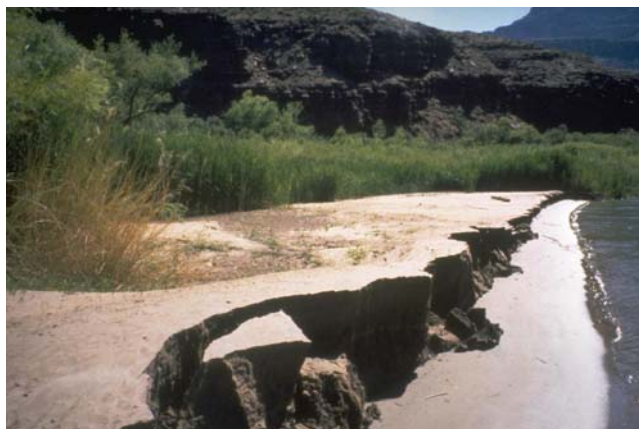
PHOTO 4- 11: BEACH EROSION AT FURNACE FLATS
