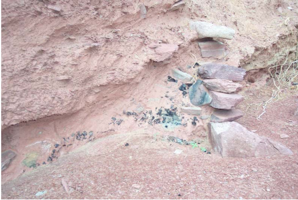
PHOTO 4- 9: EXAMPLE OF EROSION AT A SIDE CANYON SITE
