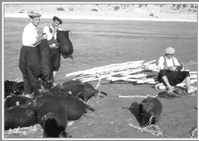
First things first: assembly of the boat begins with inflation of the "tubes" - actually complete sheepskins sewn together to be both water tight and air tight, and the fabrication of a wooden frame.
